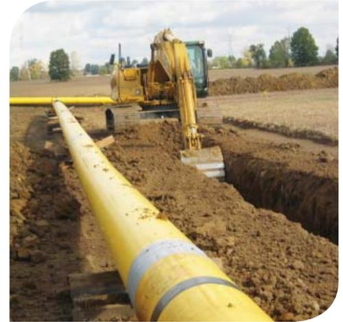
*It is becoming more common for pipelines to be constructed within existing AC transmission corridors. While this approach addresses many challenges typical of new pipeline construction, AC interference can present additional safety and corrosion-related issues.*
